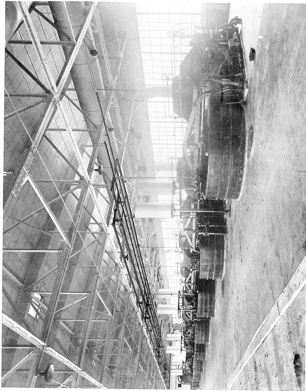
THE BEATER ROOM OF K. V. P. MILL NO. 2 Where rags are made into the clean, pure "stuff" which is the foundation of all K. V. P. Products
